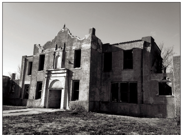
Mosheim School - Img Courtesy of Toby Petzold
